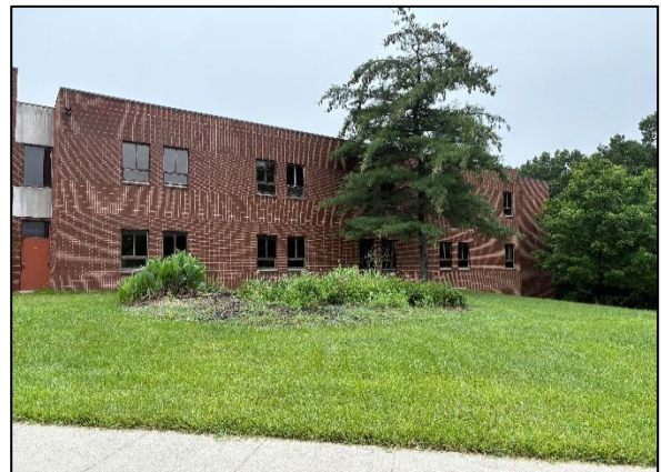
Figure 1. CTPHC exterior, June 2025.
